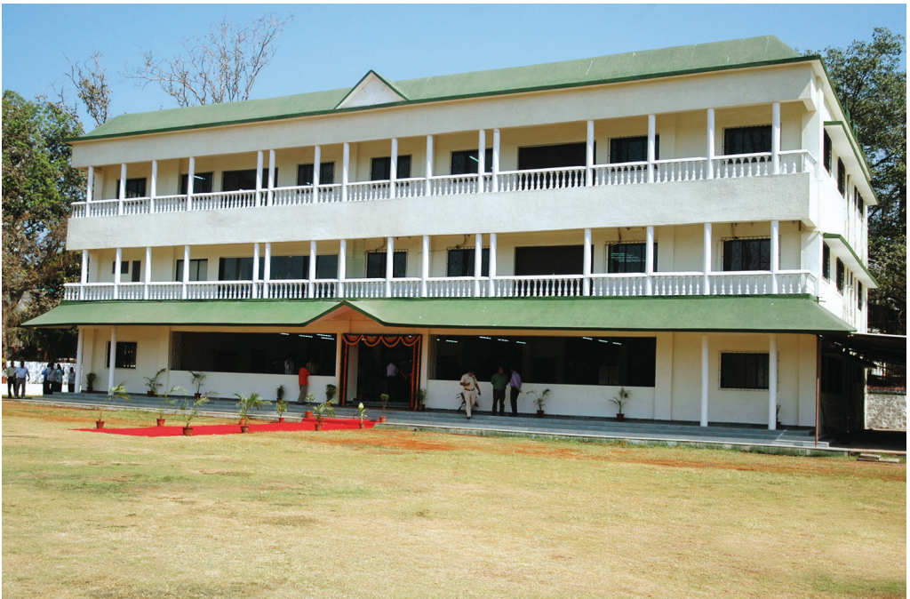
Staff Hostel at Mahalaxmi Western Railway
