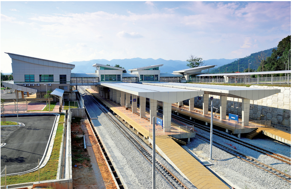
Rembau Station Building of Seremban-Gemas Electrified Double Track project by IRCON, Malaysia
