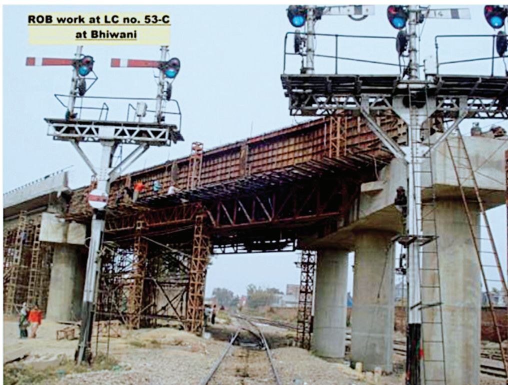
A view of Construction of ROB on North Western Railway
