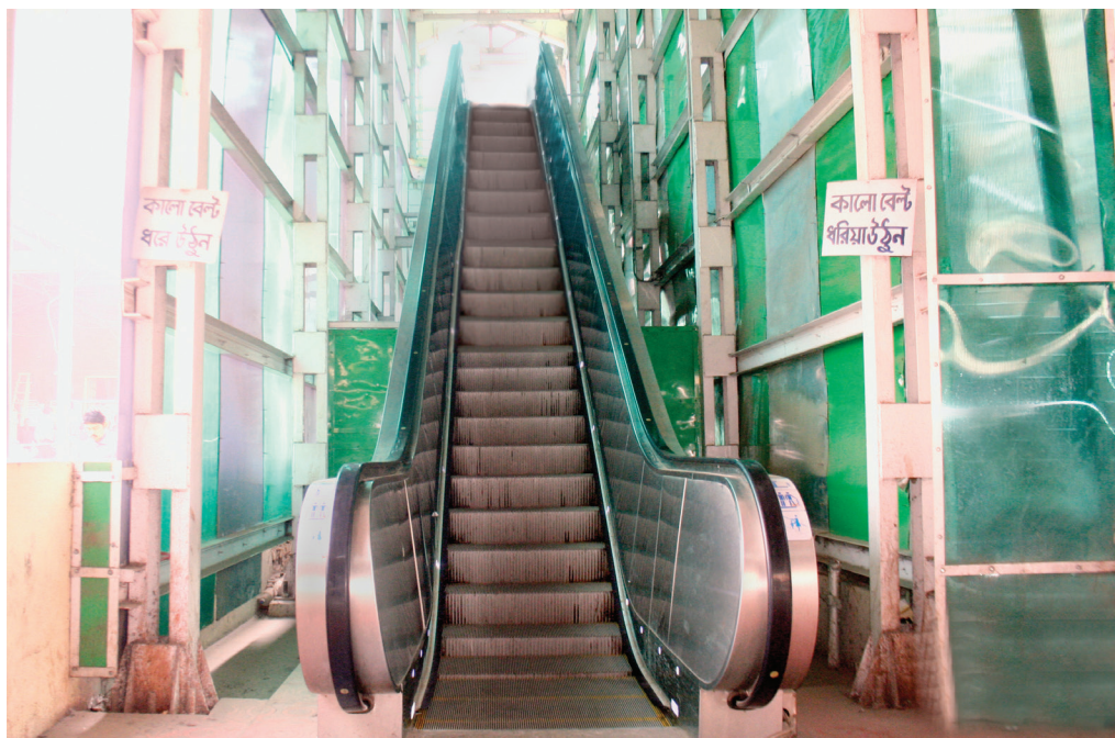
Escalator at Howrah Station, ER
