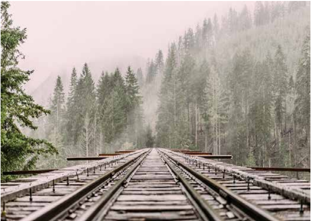
Panoramic View of Newly built track
