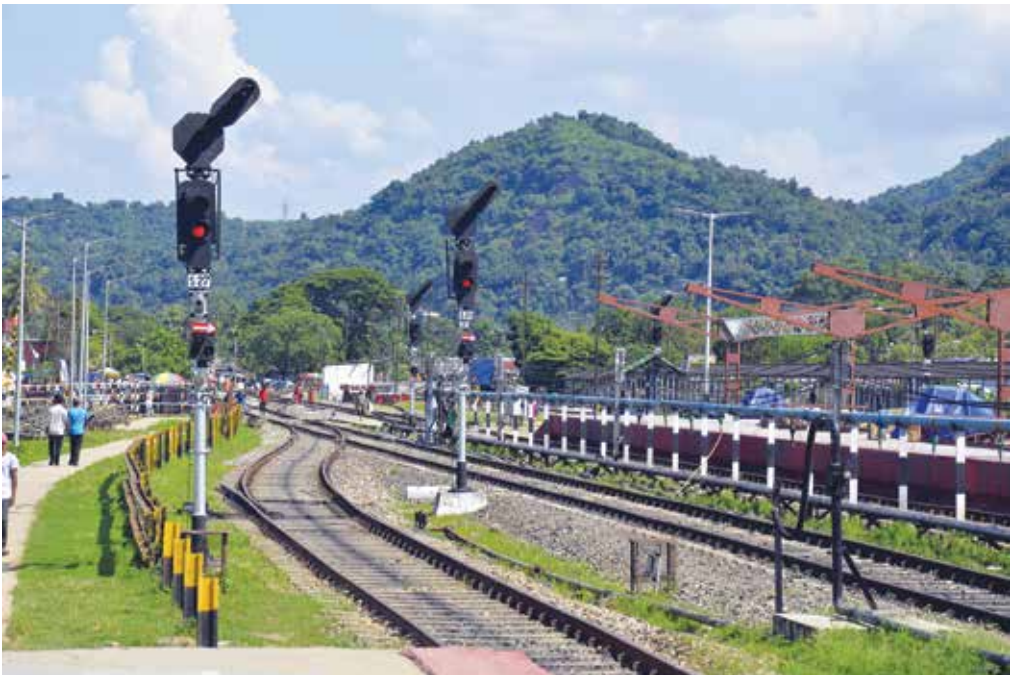
Signal & Safety Devices at NF Railway
