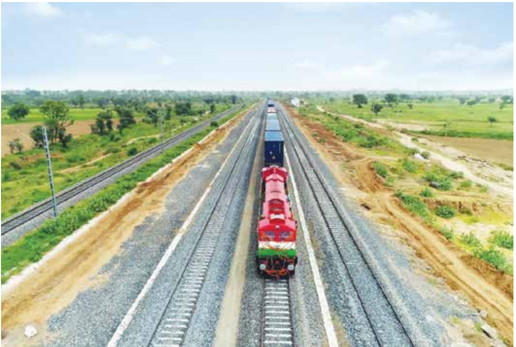
Aerial View of the Double Stack Freight Train during the trial run on WDFC's Ateli- Phulera sections on 15.08.2018.
