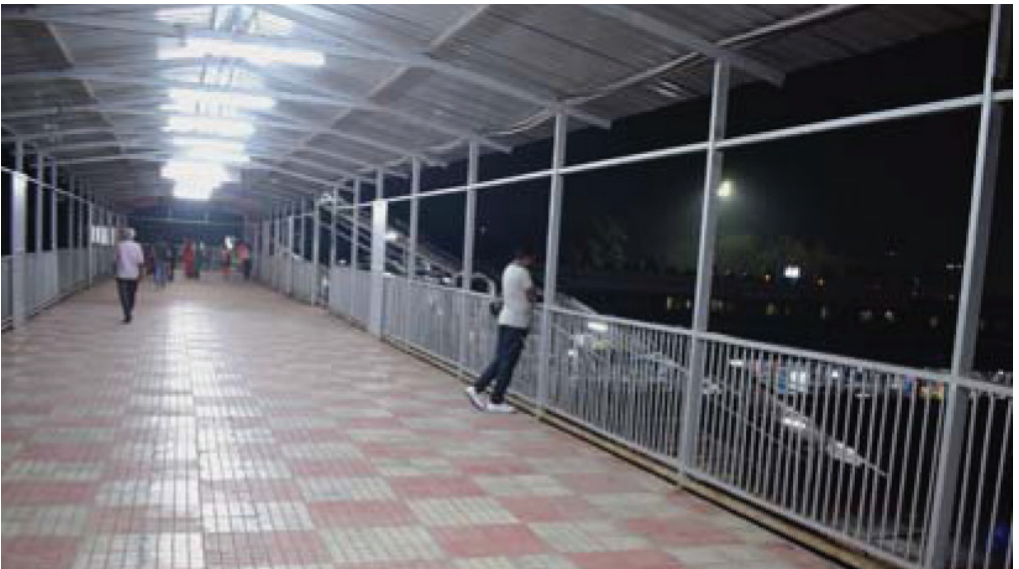
Railway Foot Over Bridge at Ranchi Station South Eastern Railway
