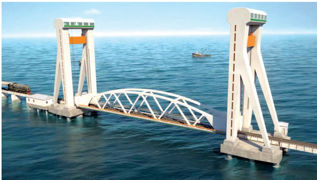
Pamban Vertical Lift Bridge an Engineering Marvel through an Iconic Bridge
