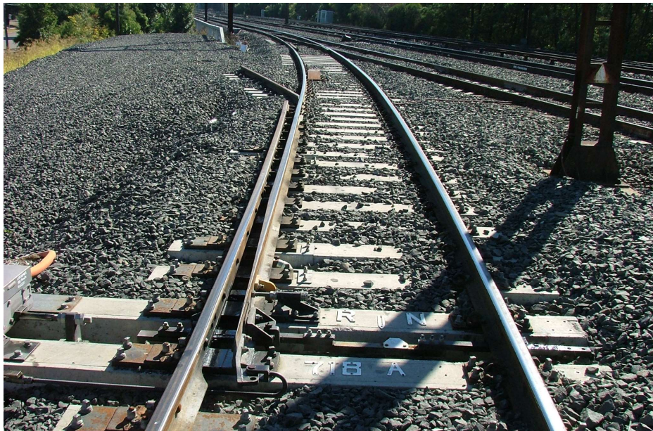
Figure 4 – Example of catchpoint with good landing zone
